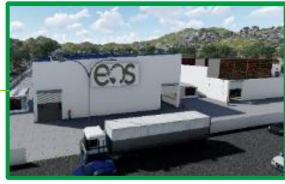
Containerized Power House
